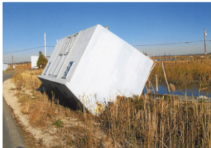
Toppled shed in Delaware Bay marshland
