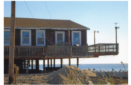
Suspended deck of beach house in Fortescue, NJ
