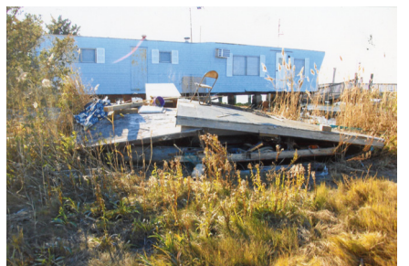
Remnants of a deck along the Delaware Bay
