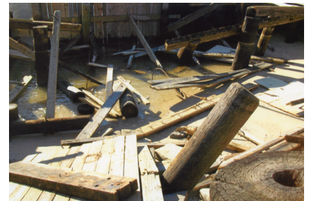
Ravaged deck of Charlesworth Restaurant, Fortescue, NJ
